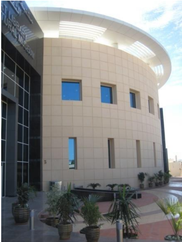
Main Entrance and Landscape
